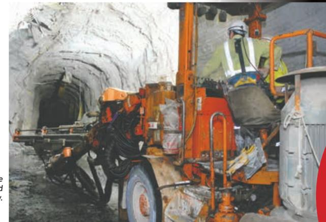
Five metre by 5 metre tunnels will be constructed to access the orebody.
