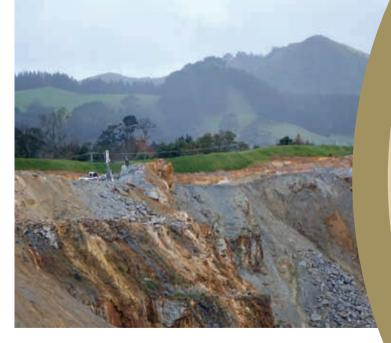
radar system and other devices. The radar has provided important accurate information at every stage of the project. You can see the white radar dish from the viewing area near the Cornish Pumphouse. It is pointing across the open pit towards the North Wall. The company will continue to monitor and further stabilise the north wall if required to mitigate any further issues.
