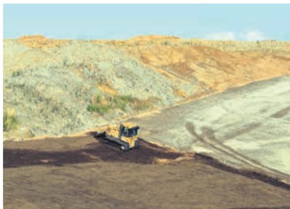
Above left: Topsoil being spread on the top of the tailings impoundment. The area to the right has just been fertilized with lime.
