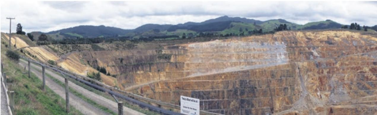
Soon, instead of pushing the material down into the pit we will be trucking it to the ROM pad next to the crusher then transporting it to the Development Site on the conveyor.
