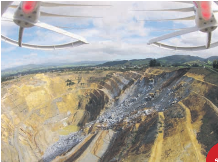
This photo was taken with our quadcopter a few hours after the rock fall. It clearly shows the amount of material that has fallen out of the wall and how much is in the bottom of the open pit.
