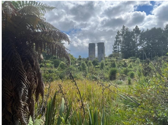
Figure 12 Decommissioned cyanide tanks at Union Hill with native planting in the foreground
