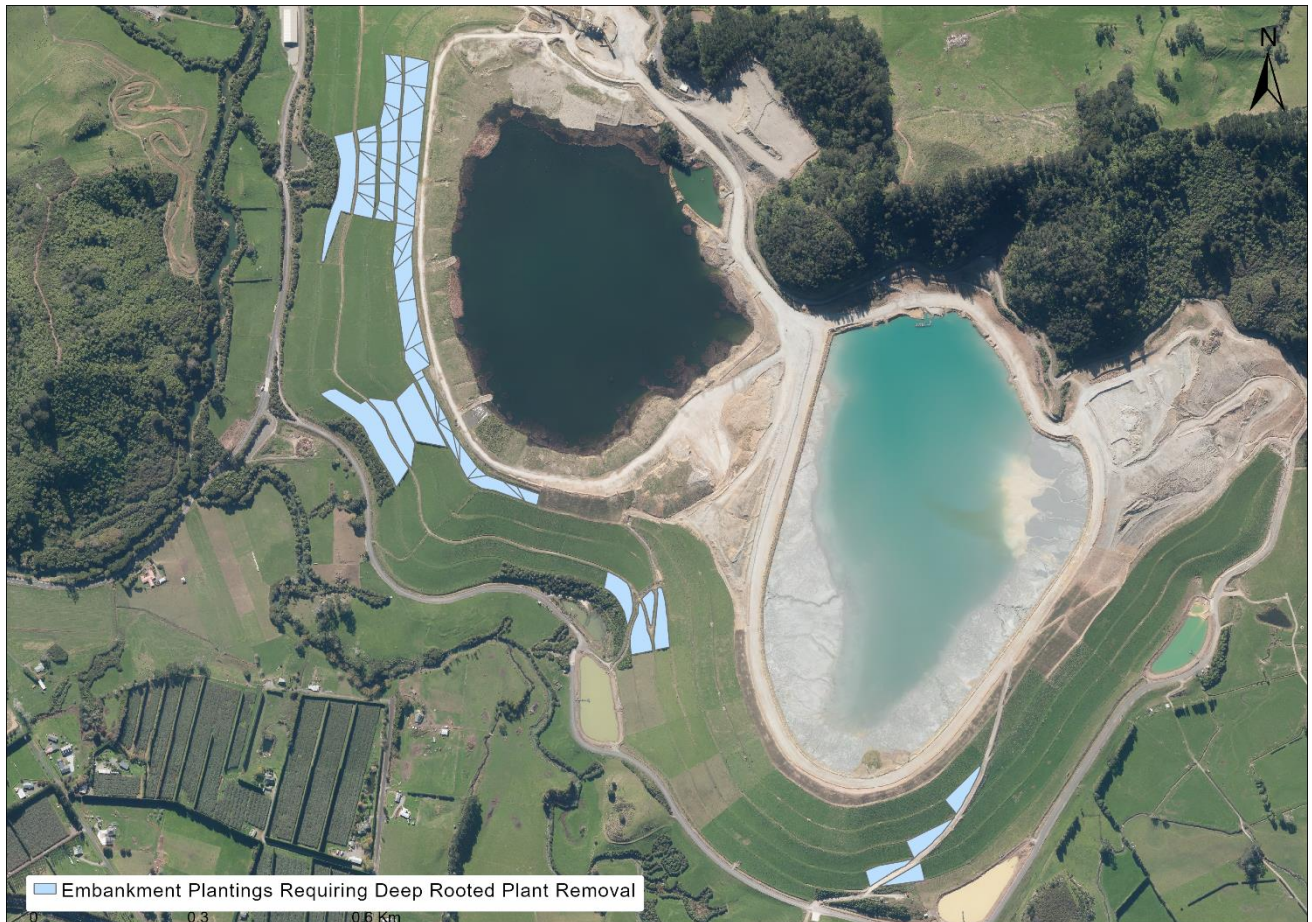
Figure 16: Embankment Plantings Requiring Ongoing Deep Rooting Tree Removal
