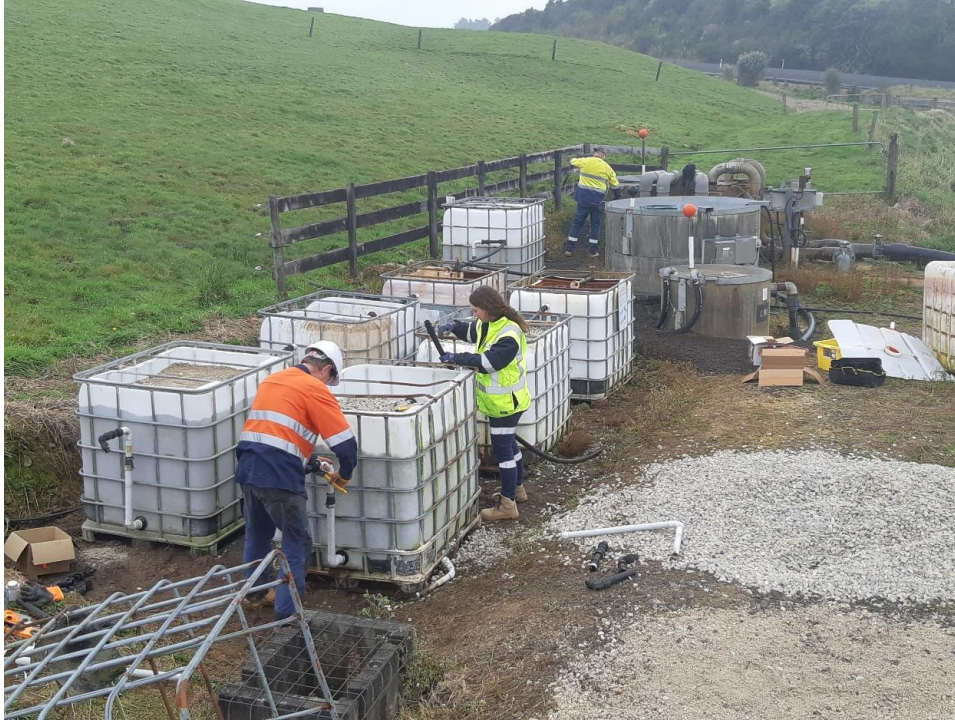
Figure 17 Installation of passive treatment trial at TU site.
