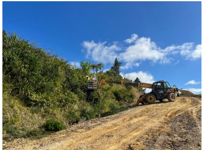
Figure 34 Telehandler operating at the SW end of the Pit to access hard to reach areas safely.
