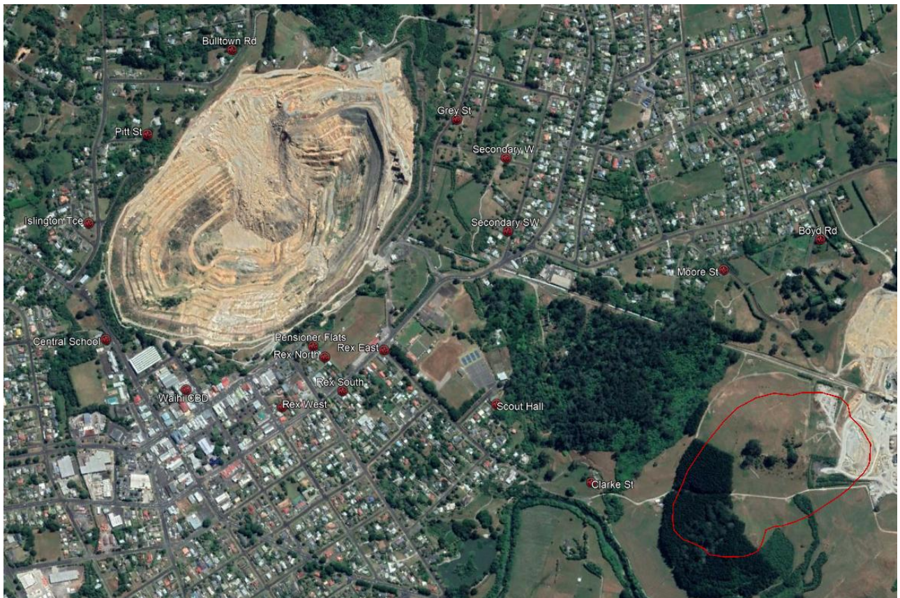
Figure 2 – Fixed Vibration Monitors for Martha Pit and Underground and for GOP
