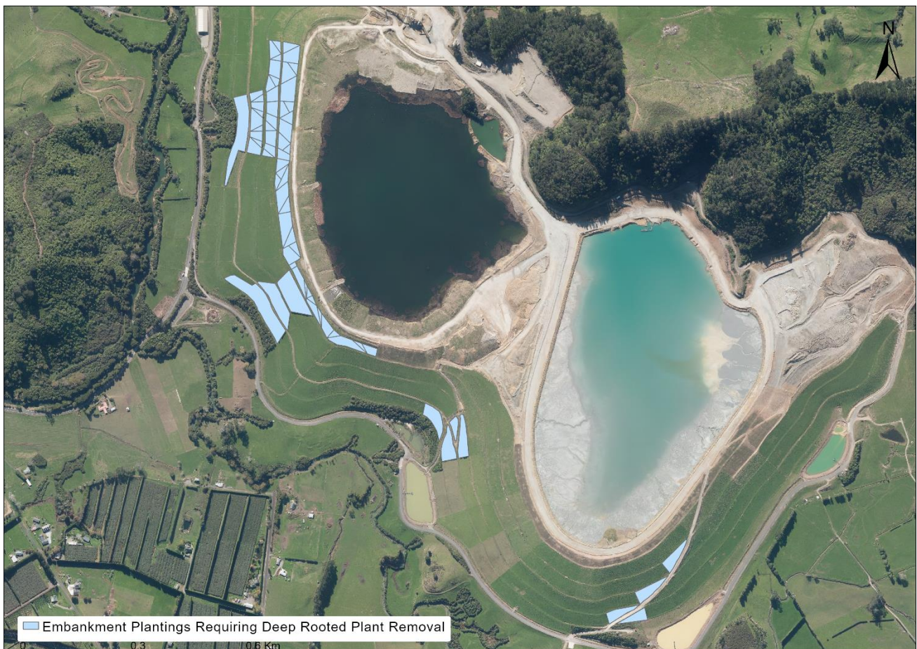
Figure 9: Embankment Plantings Requiring Deep Rooting Tree Removal
