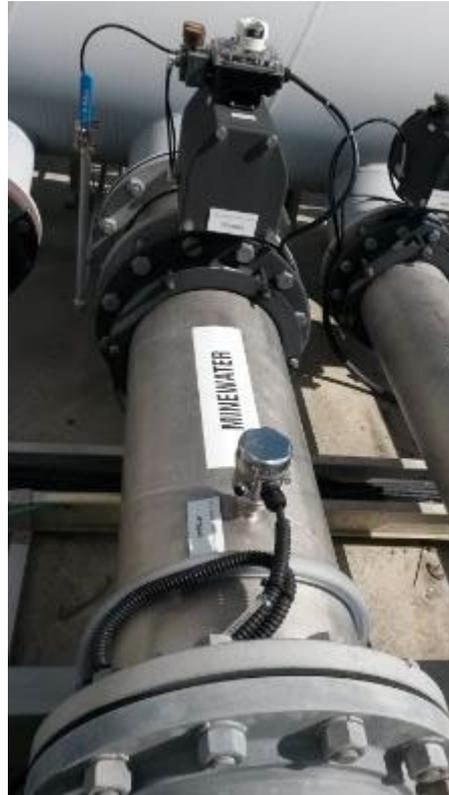
**Figure 4: Underground dewatering sample spigot**
