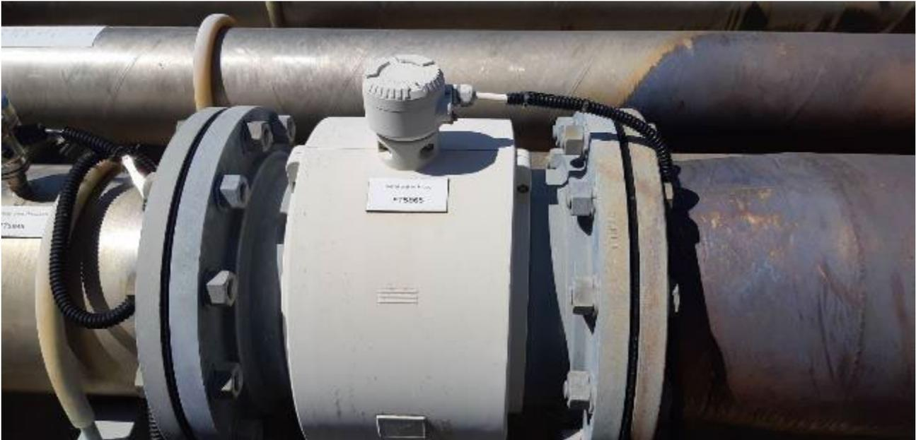
**Figure 3: Dewatering totalising flow meter**
