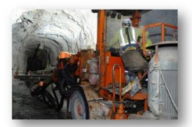
Left: A development drive. These drives are tunnels five metres high by five metres wide, carved out of the rock by drilling and blasting. The ceiling and walls of the drive are bolted and meshed before being sprayed with concrete. Electric power, water and compressed air lines also run inside the drive. Drives like this one provide access to the ore body.
