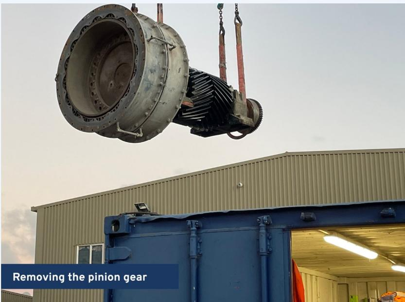
Removing the pinion gear
