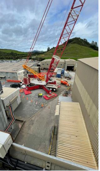
As part of our processing plant upgrade, we're currently working to remove our old SAG mill to replace it with a new one. Due to its weight and size, we had to remove the mill in pieces through the roof of the building. This involved removing the girth gear in two halves (17.5-tonnes each), discharge head and feed head (38-40-tonnes each), main mill body (40-tonnes), load cell top section (9-tonnes) and the pinion (drive) gear shown above.
